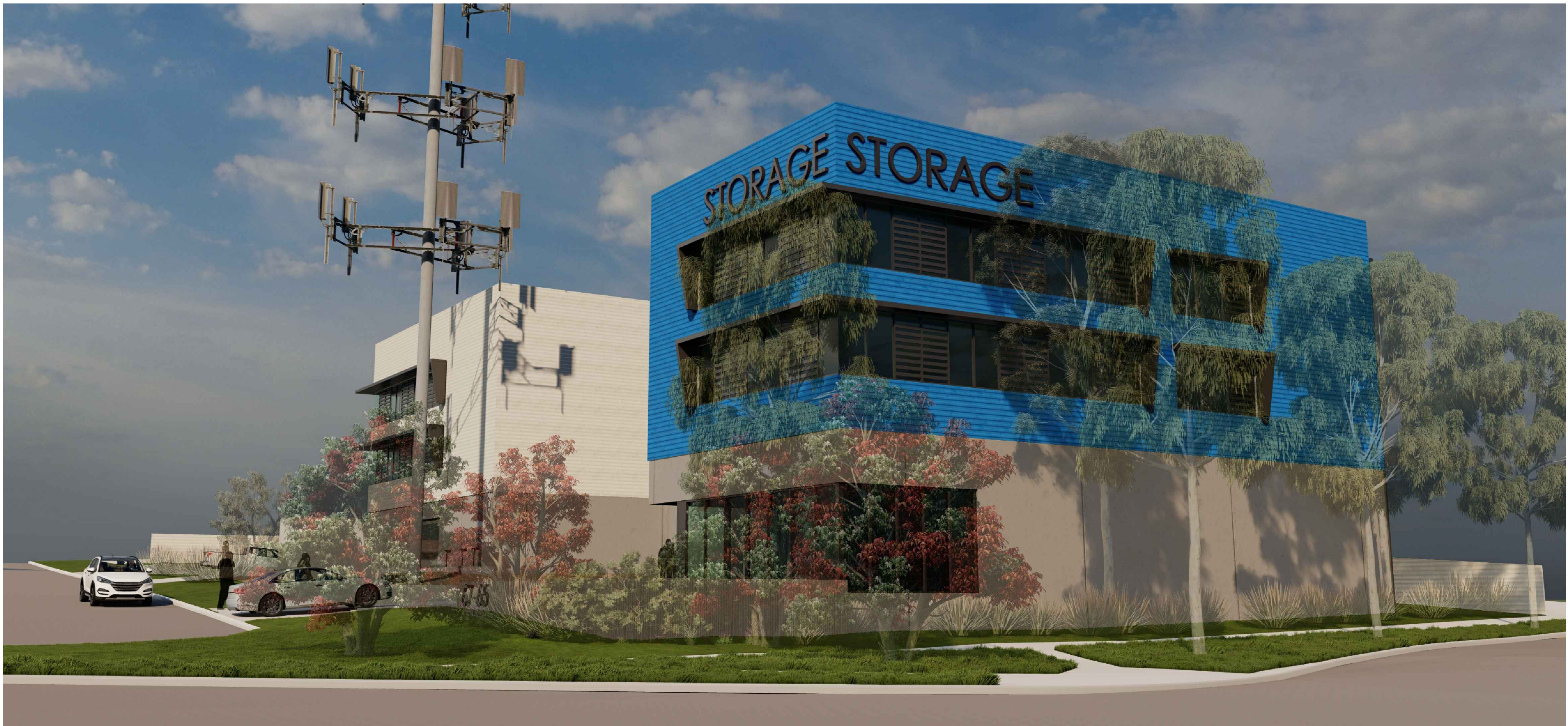
01 NORTH WEST FACADE
